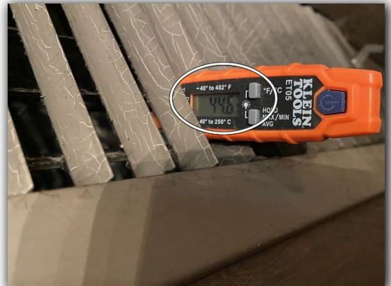
Supply air / differential
