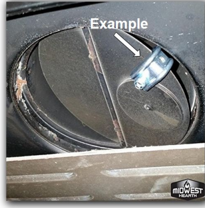
Example of damper clamp
