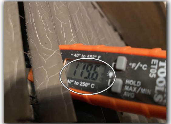
Supply air / differential
