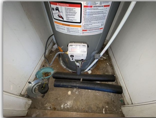
0 PPM found with CO and gas meters at time of inspection
