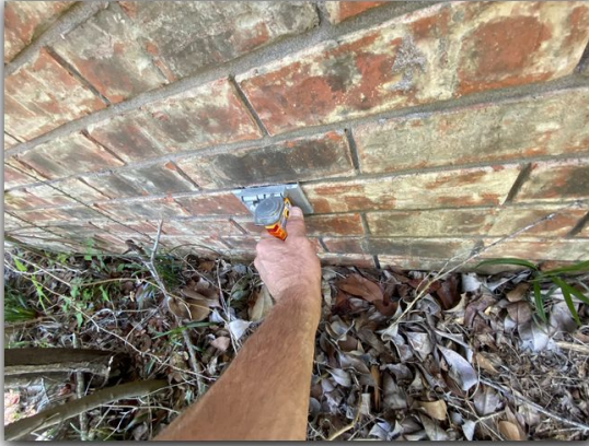
Missing GFCI protection on exterior of home
