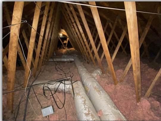
Views of attic area
