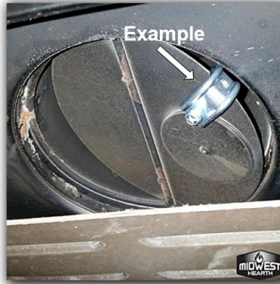
Example of damper clamp
