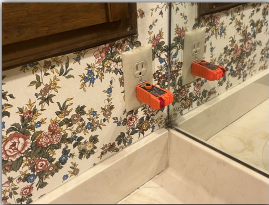
Missing GFCI protection in bathrooms
