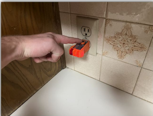
Missing GFCI protection in kitchen area
