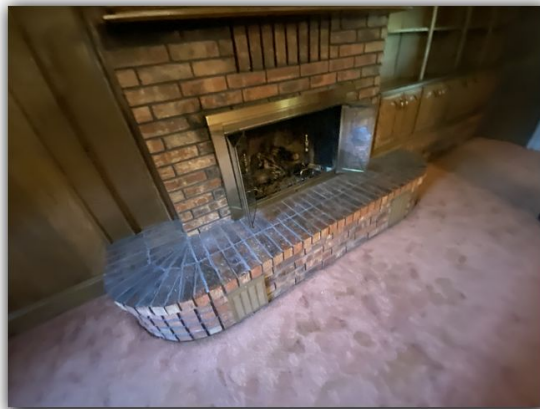
Blower appears to be working as should.
