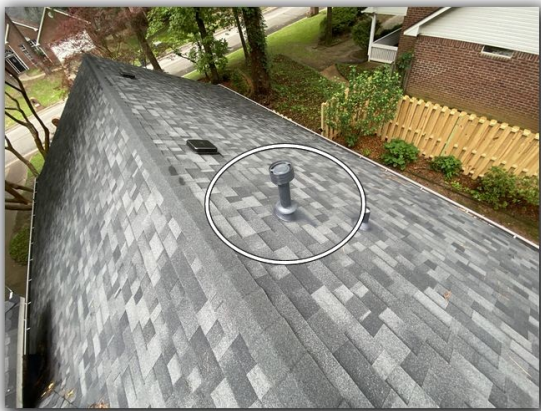
Roof area above
