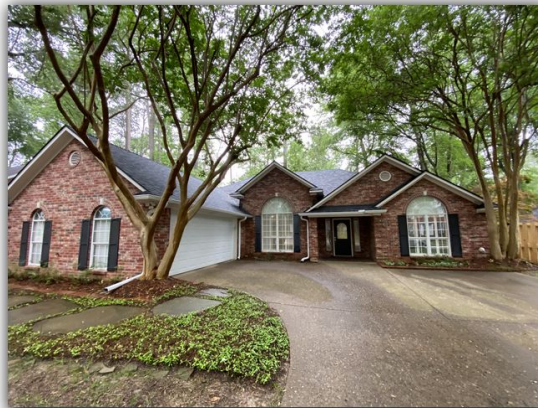
Views of exterior walls
