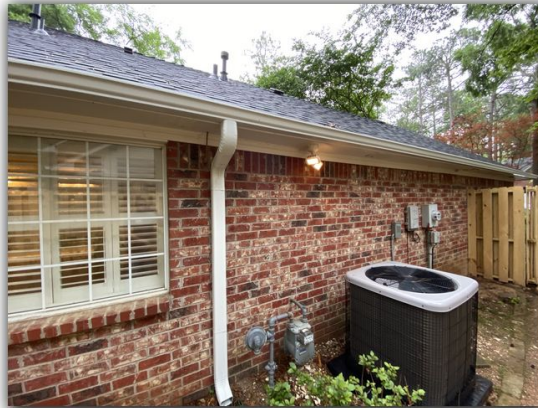
Roof area above
