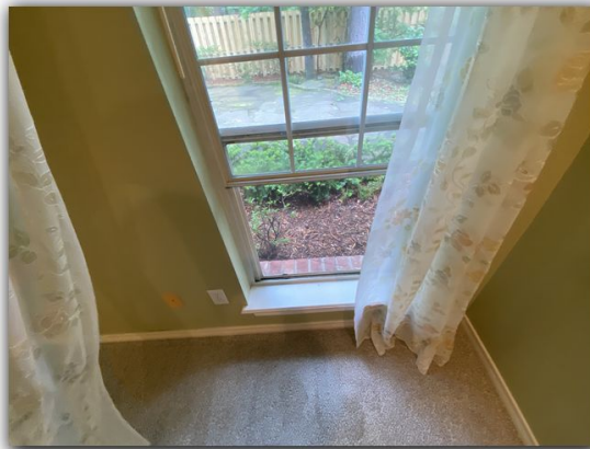
Views of windows open and operational
