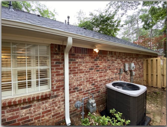
Roof area above
