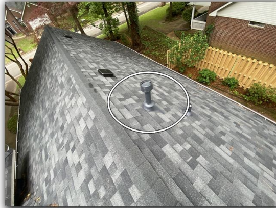
Roof area above
