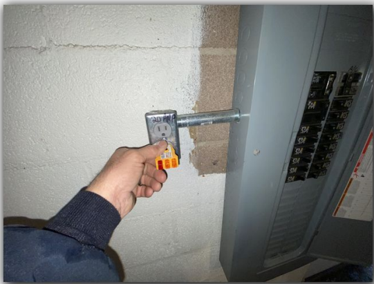
Missing GFCI protection in basement area
