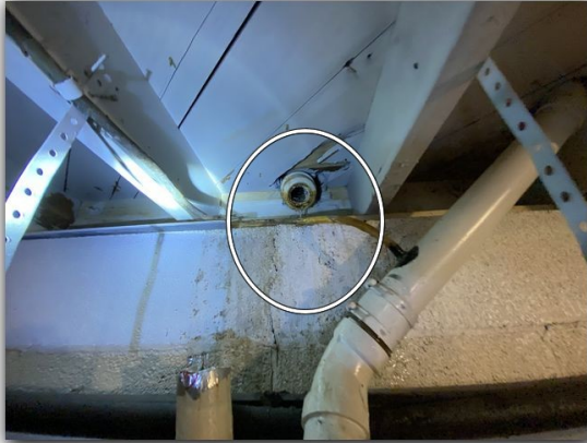
Water flowing from cut vent stack
