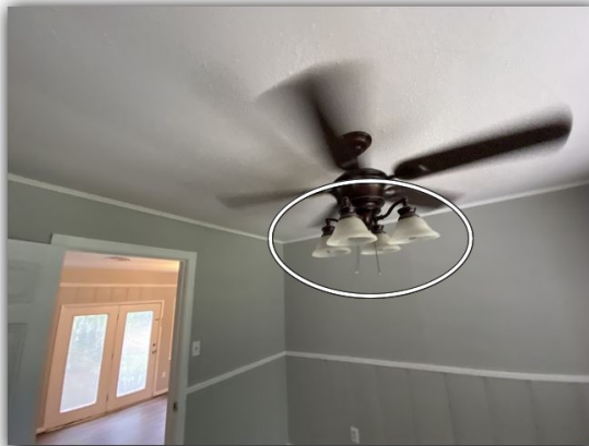
Front middle bedroom light kit would not turn on with 4 bulbs in place
