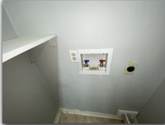
Washing machine drain
