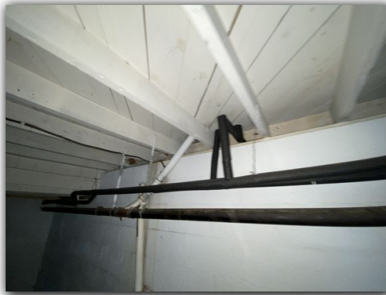
Washing machine drain
