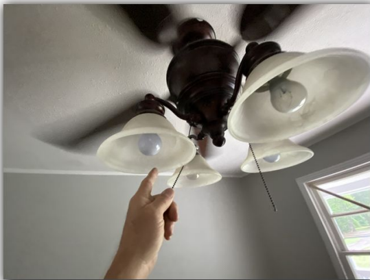
Front middle bedroom light kit would not turn on with 4 bulbs in place
