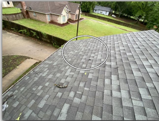
Roof area above
