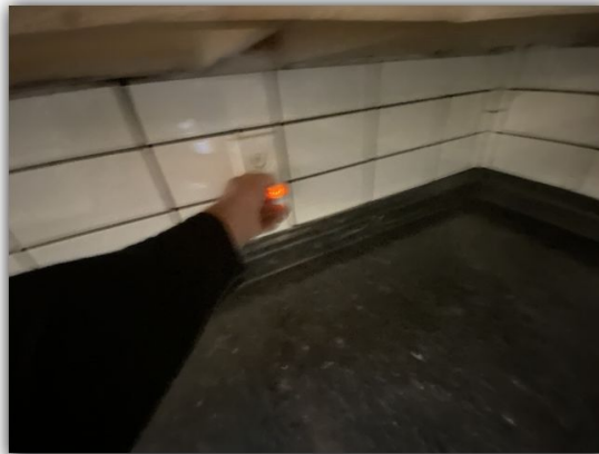
Missing GFCI protection in kitchen area
