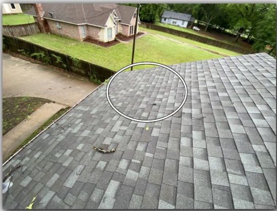
Roof area above
