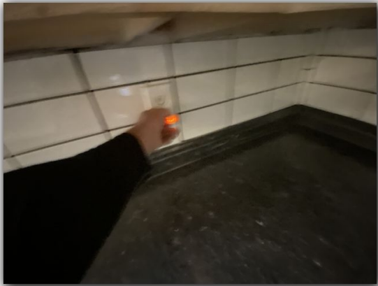
Missing GFCI protection in kitchen area
