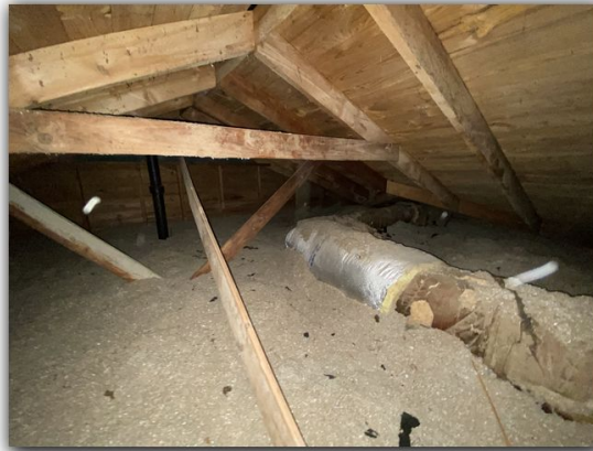
Views of attic area
