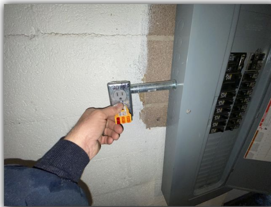
Missing GFCI protection in basement area
