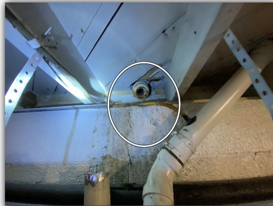
Water flowing from cut vent stack
